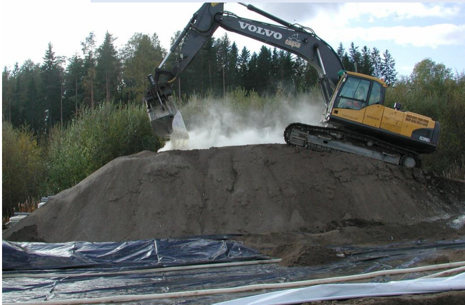
Full scale experiment about the remediation of creosote contaminated soil
