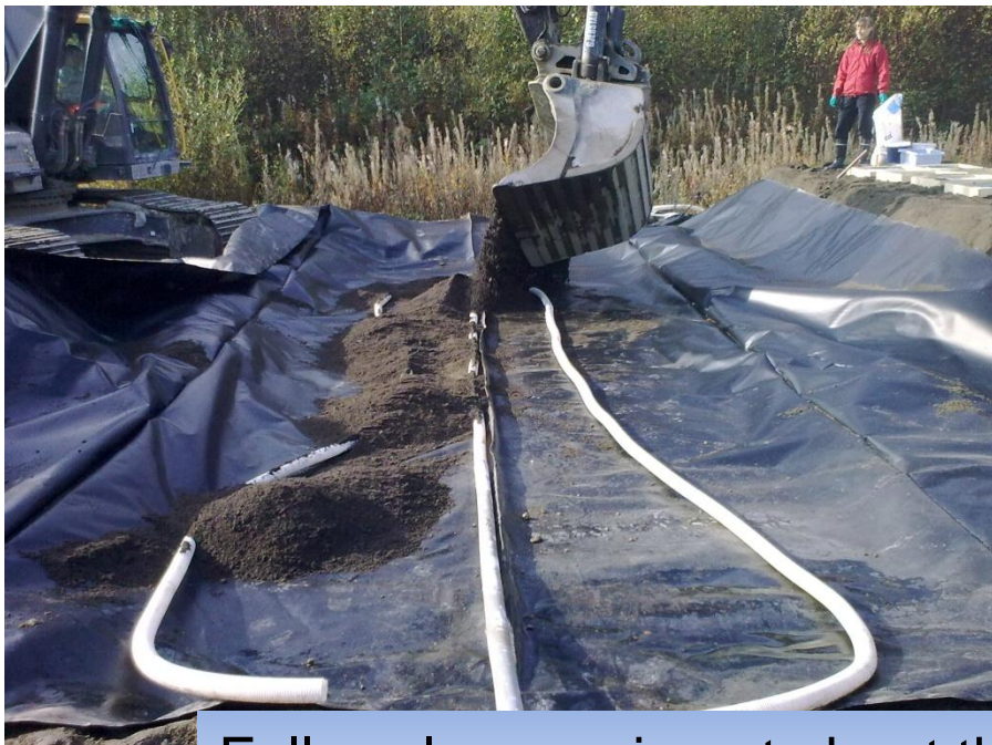
Full scale experiment about the remediation of creosote contaminated soil
